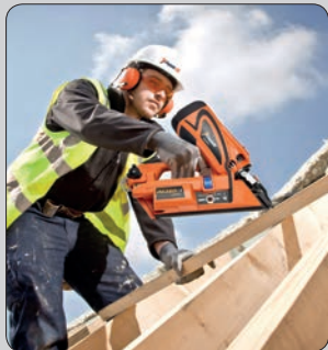
Roof battening
