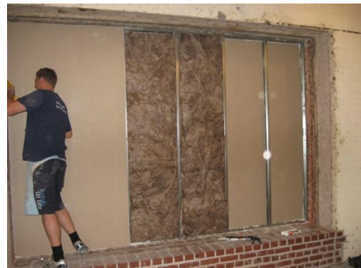
25mm thick Knauf Crown Acoustic Partition rolls
