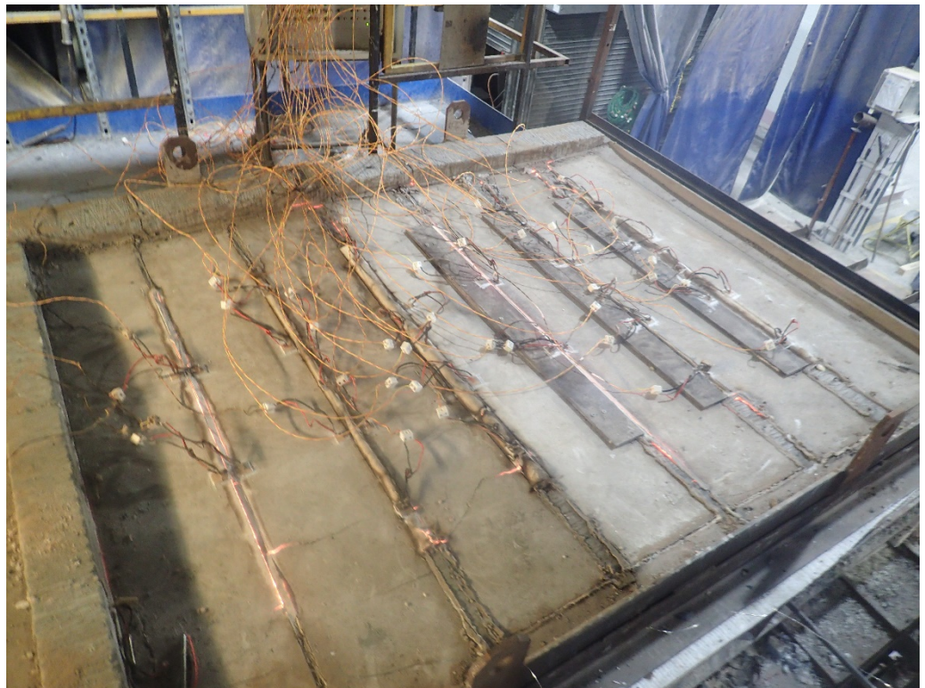
The unexposed face of the floor construction after a test duration of 264 minutes
