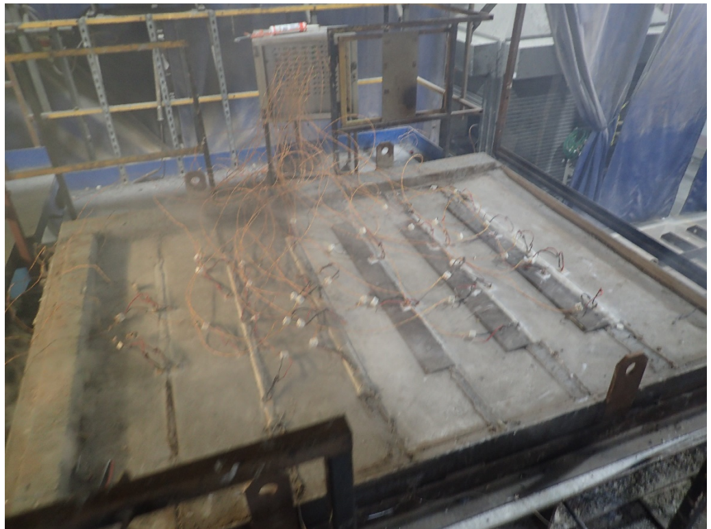
The unexposed face of the floor construction after a test duration of 71 minutes
