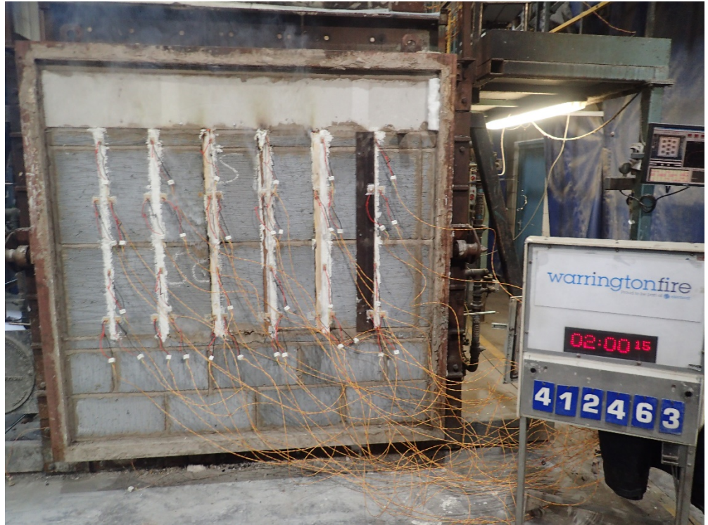
The unexposed face of the wall construction after a test duration of 120 minutes
