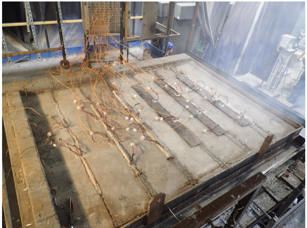
The unexposed face of the floor construction after a test duration of 120 minutes
